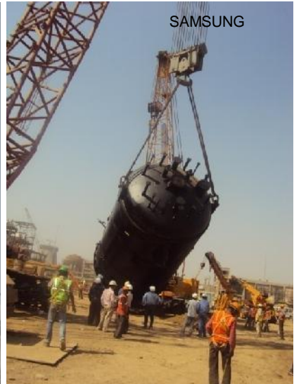
130 MT STRUCTURE MODULE ERECTION 165 MT REACTOR ERECTION AT SAMSUNG
