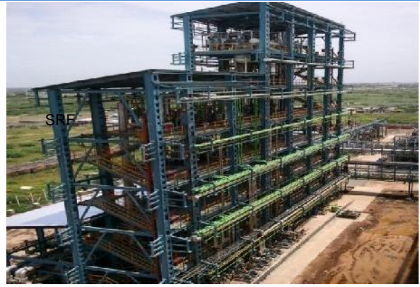
STRUCTURE, EQUIPMENT & PIPING WORK AT SRF
