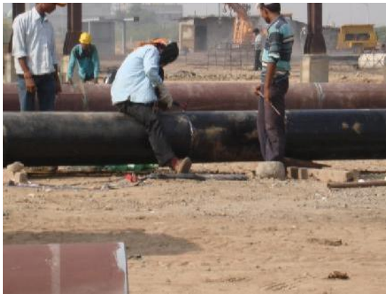
PIPING WORK EXECUTION AT MEGHMANI
