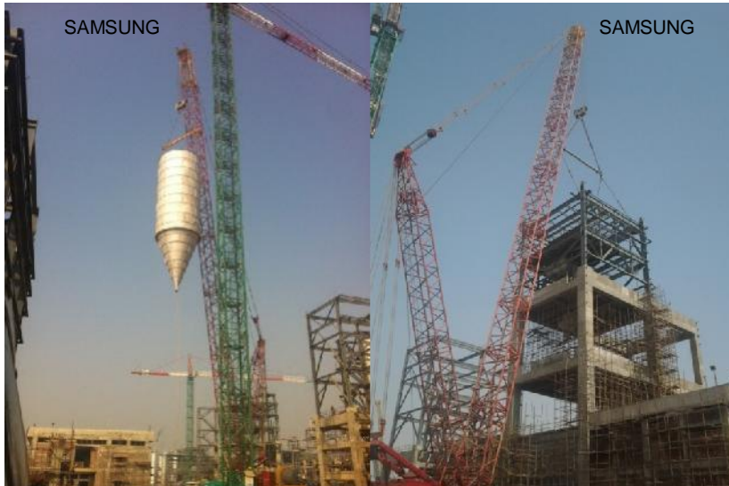
40 MT SILO ERECTION AT 52 MTR
