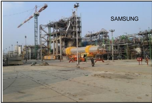
240 MT MIXER ERECTED AT SAMSUNG
