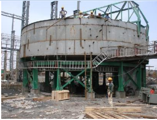
CLARIFIER FABRICATED AT BIRLA COPPER
