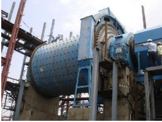
BALL MILL ERECTED AT BIRLA COPPER
